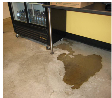
Figure 1. Spilled liquid on a floor that may cause slips.
